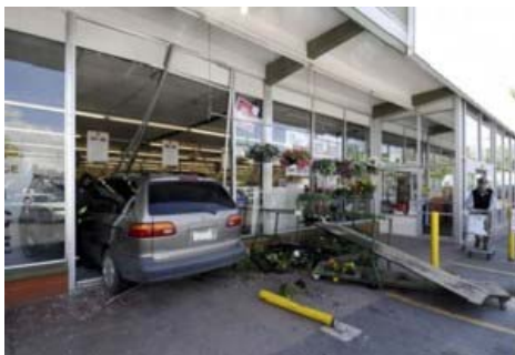
Note the failed bollard in the foreground of this storefront crash. Had the device been properly selected and installed following a qualified testing standard, this crash might have been prevented. Photo courtesy Missoulia.com.
